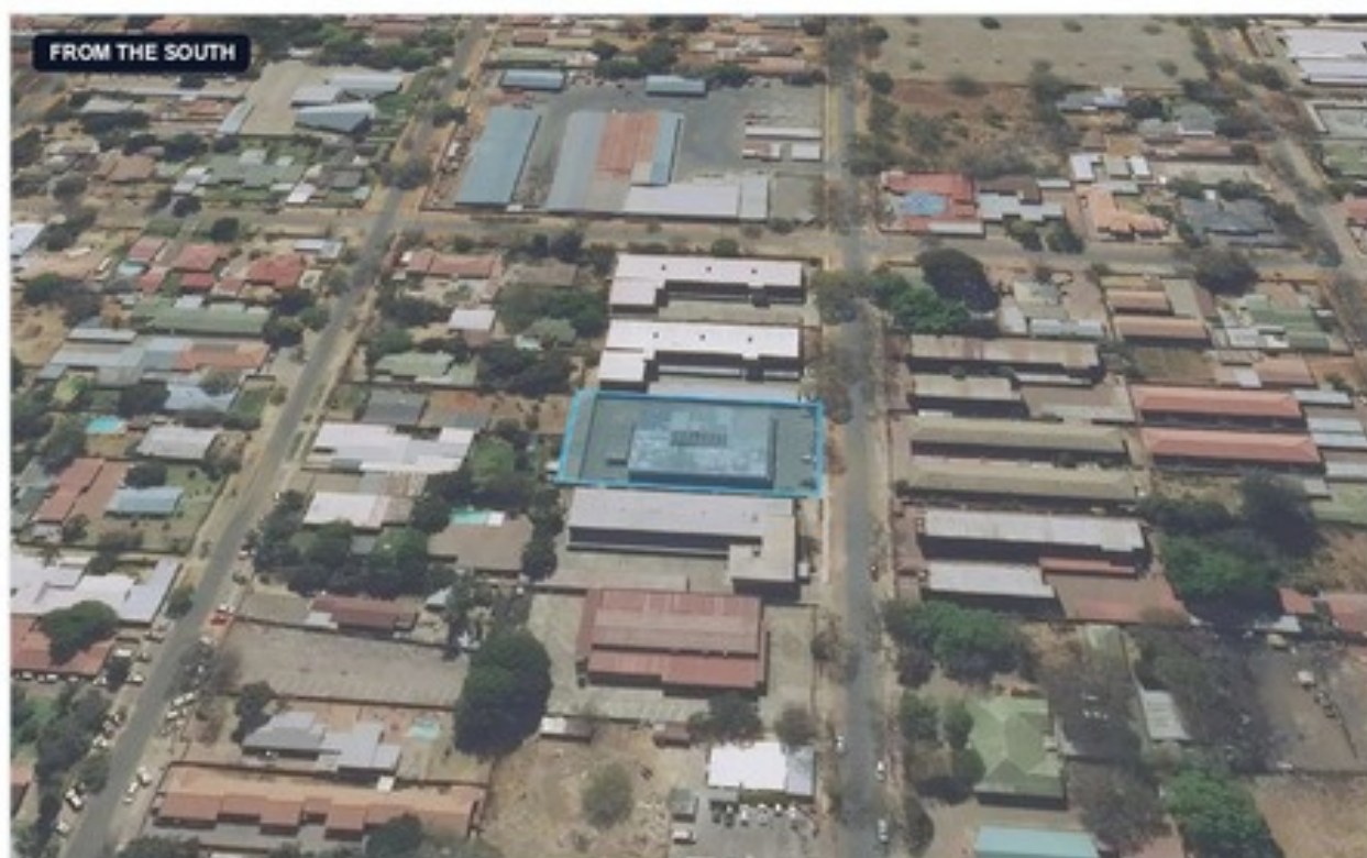
View from the south
